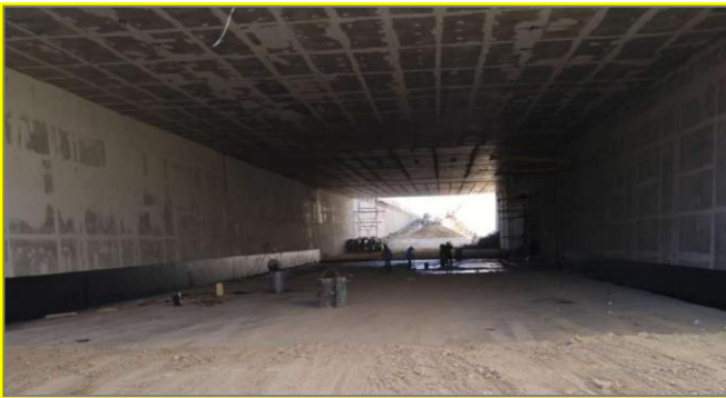
Supervising the work for the Prince Mansour Hospital tunnel in Taif 2015
