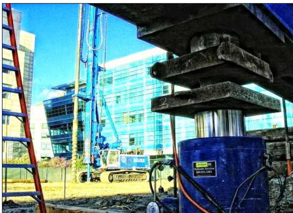
Pile Load Test
