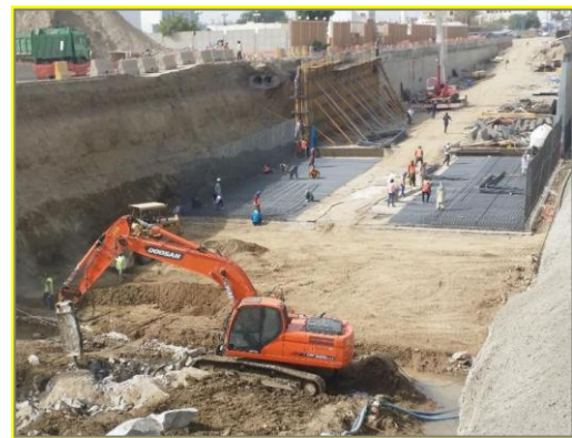
Supervising rock cut works, reinforcing works, Underpass, for the Prince Mansour Hospital tunnel in Taif 2015
