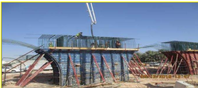
Bridge of King Fahd Road with King Abdullah Road (eastern side) in Al-Ahsa-2016
