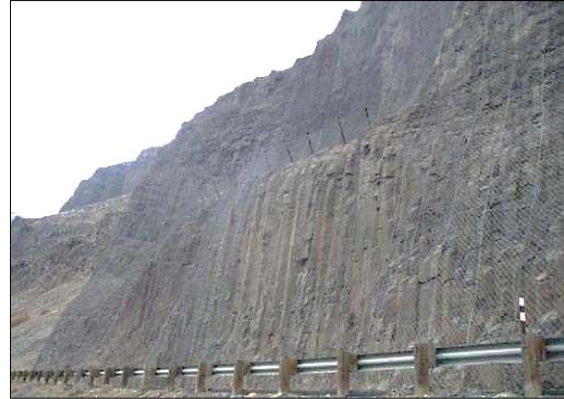
Installing rock slopes after installing a support grid
