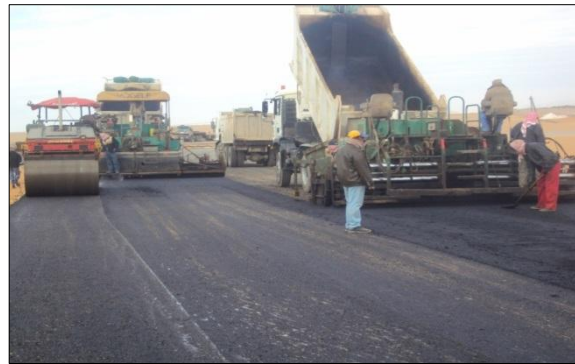
Asphalt Pavement Supervision in Arar
