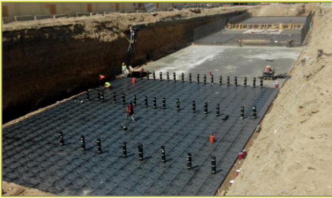
Supervising of the Concrete insulation works for for the Prince Mansour Hospital tunnel in Taif 2015
