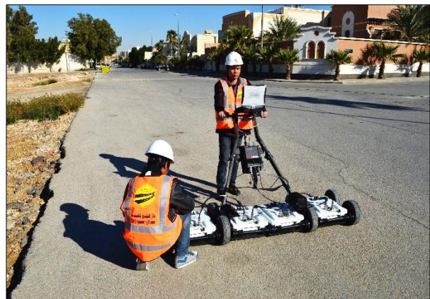
GPR Used for Utility Clearance
