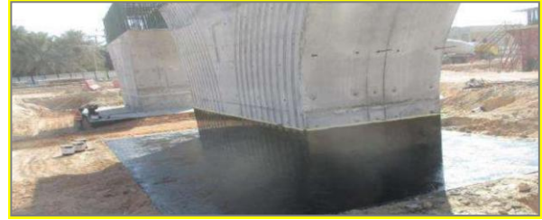
Bridge of King Fahd Road with King Abdullah Road (eastern side) in Al-Ahsa-2016
