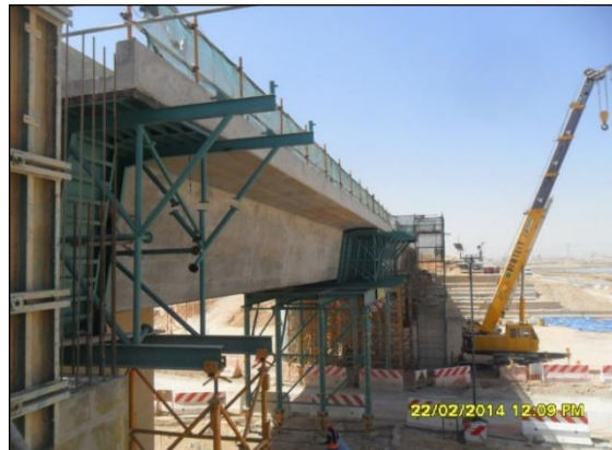
Railway track Bridge-Construction Supervision-SRO
