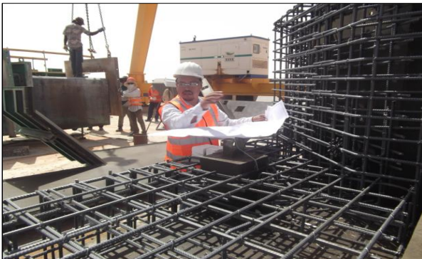
Precast Culvert Reinforcement Inspection
