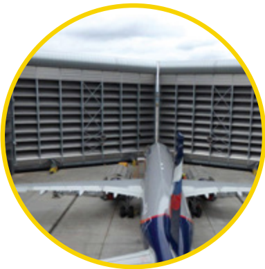
ACOUSTICALLY TREATED FRONT GATES
